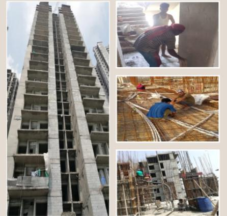
Lift brick-work, stone fixing, railing fascia casting and tile fixing work in progress • Terrace slab conduiting, tile fixing, plaster work and lintel steel binding work is in progress • Plaster work, column casting, wall steel binding and conduiting work is in progress • Villa slab casting, stair shuttering and brick step work is in progress.
