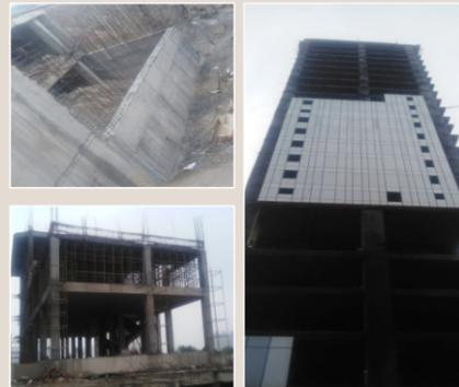
Office Tower:- Facade work in progress on 12th floor • Aluminium frame making work in progress • Aluminium section cutting work in progress • Rear Block:- Upper basement slab reinforcement binding work in progress • Non-Tower road side retaining wall casting done • Retail Block:- Ground floor staircase brick work in progress • Retail Block :- 1st floor roof slab reinforcement binding work in progress.
